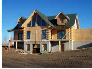
bedroom wing on the first floor. There are 9 ft ceilings on the first floor and all of the supporting and porch posts were furnished locally. Glenn had 10"-14" logs delivered and took it upon himself to hand-peel them before installation. The second floor dormer has a
